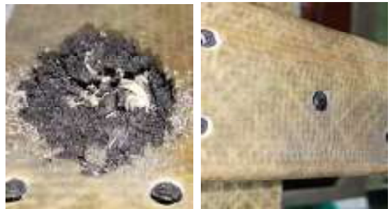
Fig. 1 FRP PIPE Surface After Drilling (Non Absorber vs Install Absorber)
